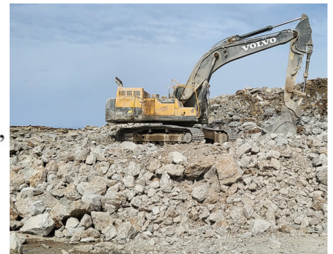
Candy Creek Crusher quarry
