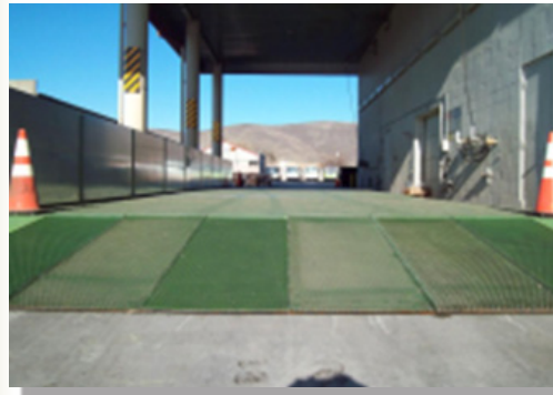
Camp Bowie Wash Platform
